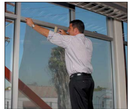
Apply to office windows
