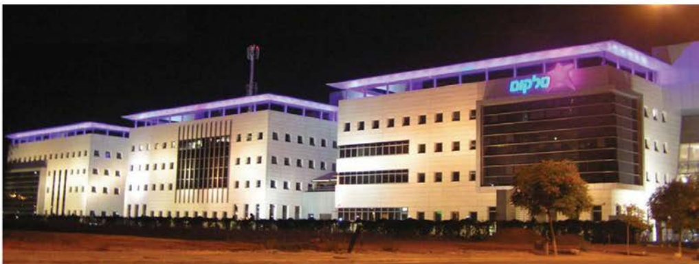
Cellcom Telecommunications, Inc. • Netanya, Israel
