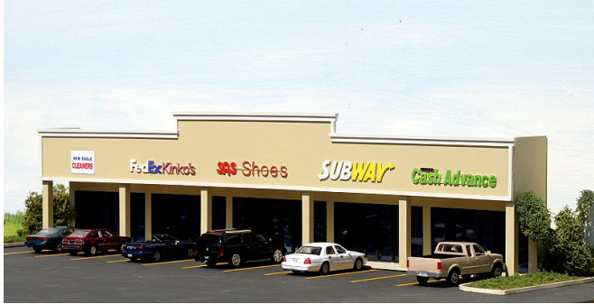
#ML-002 Strip Mall backdrop building #2
