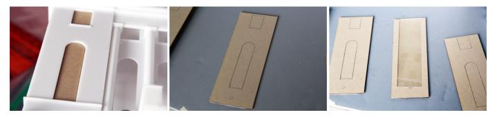
Hold the clear acrylic window glazing in place and mark the openings with a pencil, the cut away the protective paper as shown and paint it flat black.
