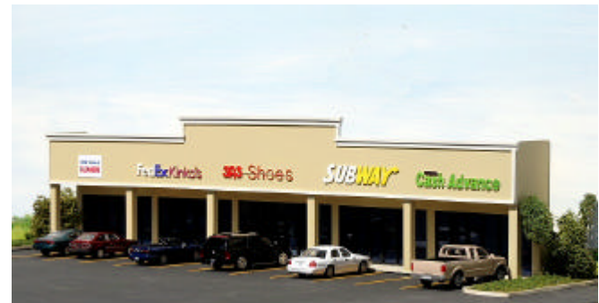
#ML-002 Strip Mall backdrop building #2
