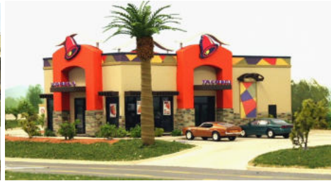
#TB-003 New Taco Bell Restaurant
