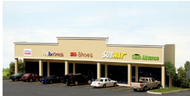
#ML-002 Strip Mall backdrop building #2
