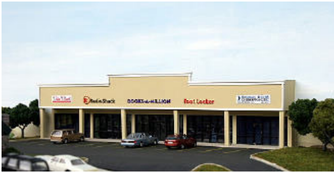
#ML-001 Strip Mall backdrop building #1
