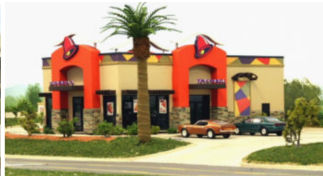
#TB-003 New Taco Bell Restaurant
