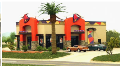
#TB-003 New Taco Bell Restaurant
