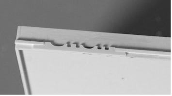
Mount the strips on the fascia. You can use the logo tool to position the strips in the correct height. Align the bottom of the tool with the bottom edge of the fascia. The logos sit on both sides of the canopy perpendicular to the street and at the end closest to the street.
