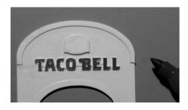
If you chose to paint the logos before mounting - after the paint has dried, you should carefully touch up the small connectors between the letters with the wall color, using a fine brush.
