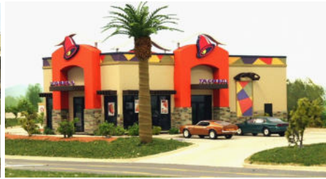
#TB-003 New Taco Bell Restaurant
